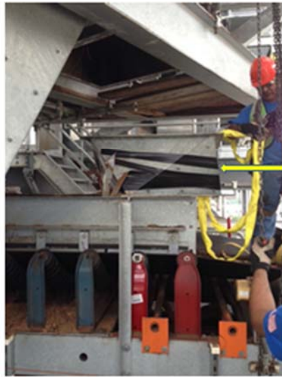
#10 conveyor chute removal
