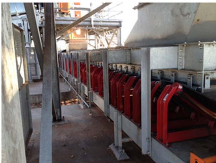
#4 conveyor belt new rollers
