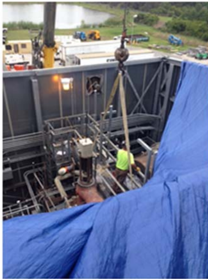
Siemens Turbine work
