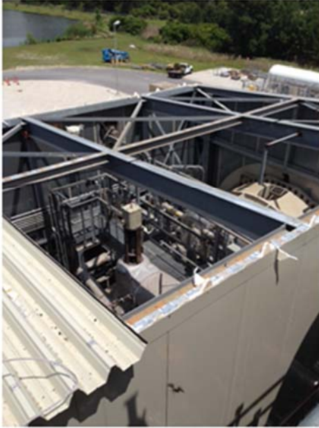
Roof removal for Turbine work
